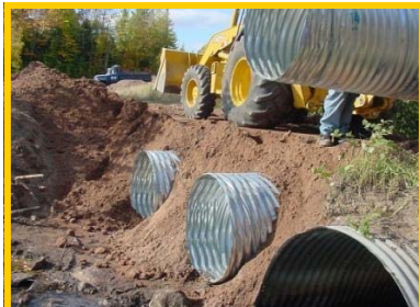
Culvert installation at Carr Lake in 2008
